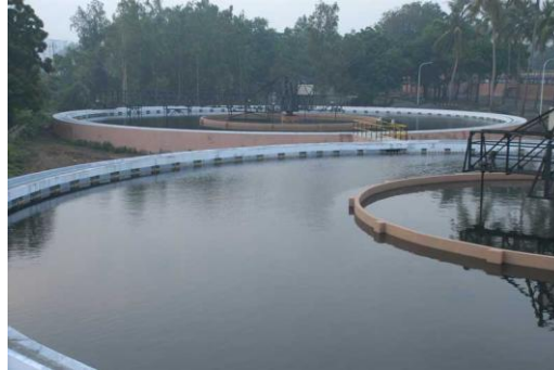
Sec. Settling Tank
