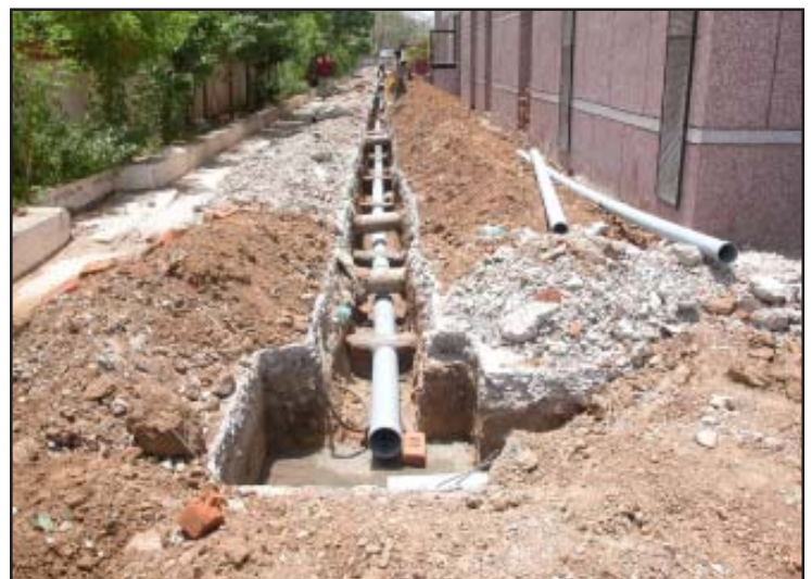
▲ 6" PVC Pipes laid in the trench
