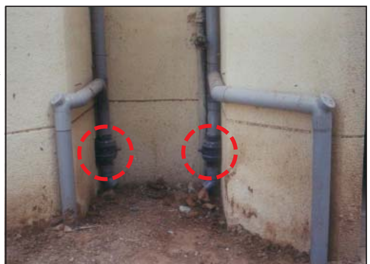
First Flush Valve fixed to the Rainwater Conveyance pipe
