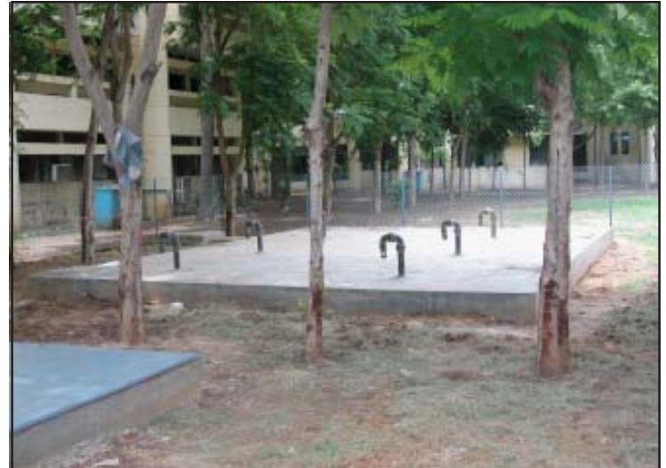
Storage Tank with Air vents ▲
