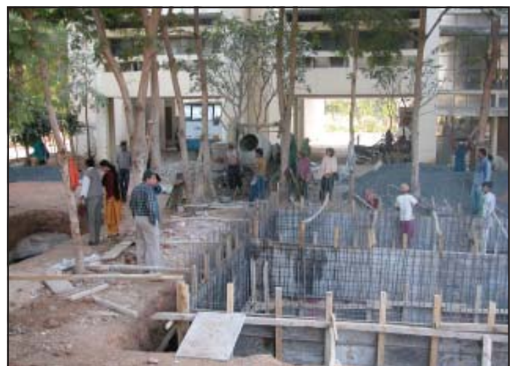
Reinforcement Steel and Shutter fixing for Storage Tank
