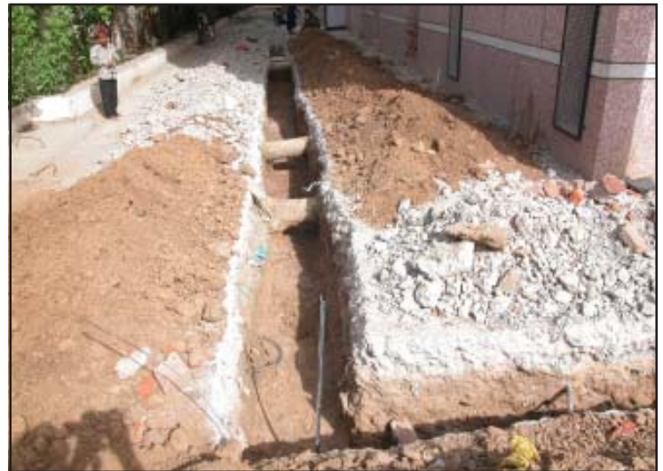
▲ Trench dug for laying PVC pipes for conveying rainwater
